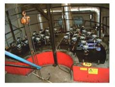
Mounting of an AEROVIT system August 2005 Before the boiler had to be cleaned 10 times/year The flue gas temperature was on a clean boiler 165°C The manuel cleaning was executed by 200-210°C
