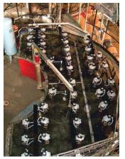
**Mounting of an AEROVIT system August 2005** Before the boiler had to be cleaned every 6. week The flue gas temperature was on a clean boiler 210°C The manual cleaning was executed by 250°C
