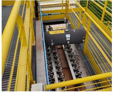
At Klabin S.A., ComBio uses wood chips and sugarcane bagasse as fuel. It is estimated that this biomass mixture would require a total stop of the steam generation plant every 3 months for cleaning the boiler pipes.
