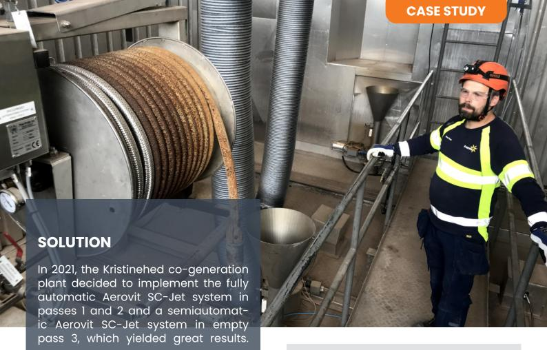
The frequency of soot cleaning in the empty passes decreased from 3 times per day to just 3 times per week which saved 86% of water. In addition they experienced noticeable drop in average flue gas temperature by approximately 65°C.
