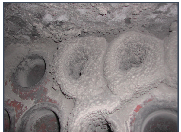
soot accumulation in a biomass boiler
