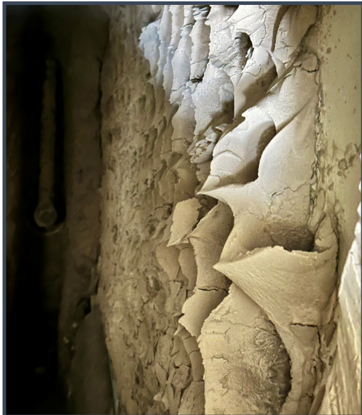
Soot and ash buildup at the tube plate
